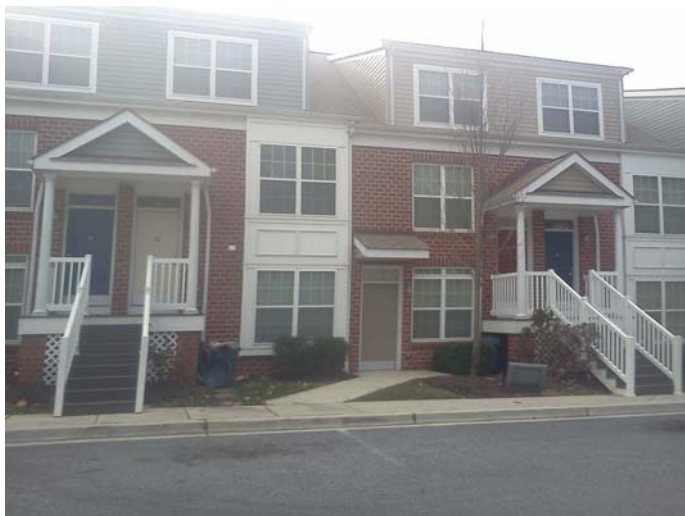
Figure 11: Constructed Buildings for Obery Court
